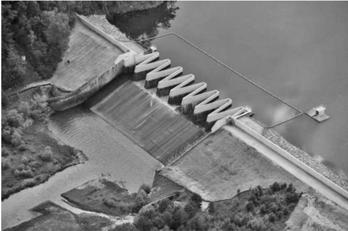
Figure 2. Example of a labyrinth type spillway with no stilling basin or plunge pool, image from Crookston and Tullis (2013).
